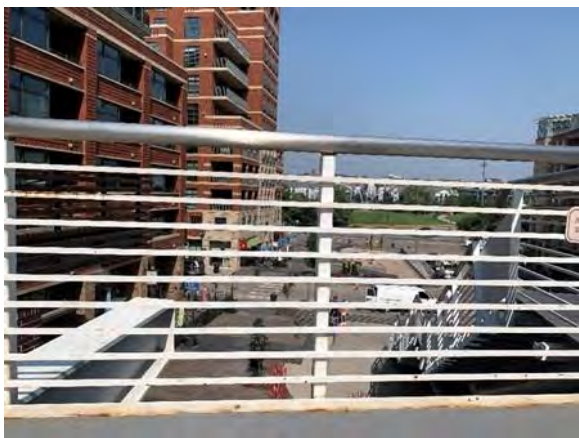
Typical Condition of Pedestrian Railing
