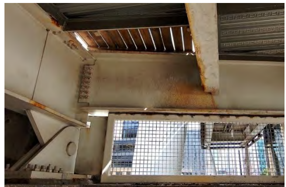
Superstructure Below City Side Elevator Platform
