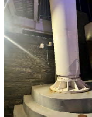
Figure 18 – Abandoned upright floods
