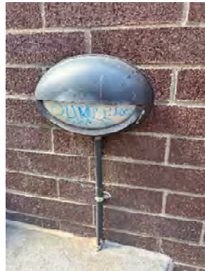
Figure 14 – Steplight with graffiti on lens
