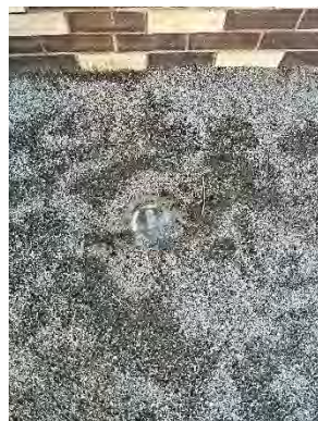
Figure 1 – Partially Covered Wallwash
