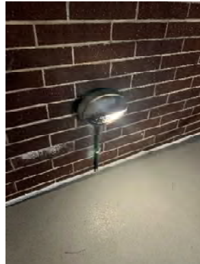
Figure 12 – Steplight with black substance on lens
