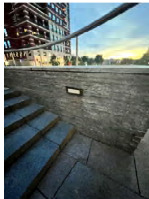
Figure 3 – Parkside non-operational steplight
